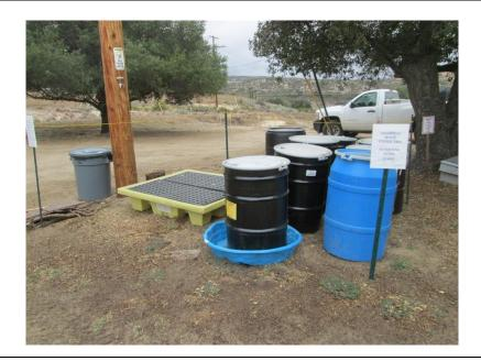
**Photo 2:** Hazardous materials are securely stored with secondary containment and labeled in accordance with Mitigation Measure HAZ-1A and the Hazardous Materials and Waste Management Plan at the Boulevard Substation Rebuild site.
