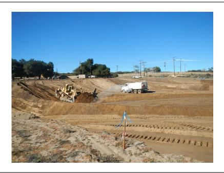
**Photo 1:** Water trucks are utilized on a regular basis to minimize fugitive dust emissions in accordance with MM-BIO-4A and the Dust Control Plan at the Boulevard Substation Rebuild site.
