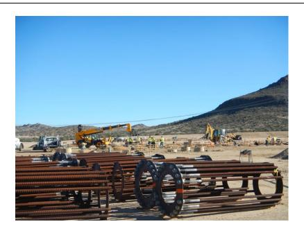
**Photo 3:** Construction crews completing concrete foundations for the control and maintenance shelters at the 138/230 kV ECO Substation pad.
