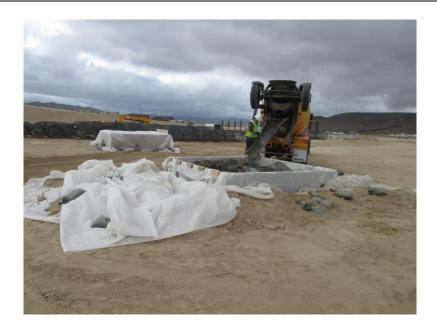
**Photo 4:** A concrete washout basin is being utilized for washing out concrete trucks following foundations pours at the 138/230 kV pad site in accordance with the SWPPP and MM-HYD-1.
